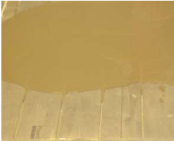
Application of Ultraplan Renovation Screed
